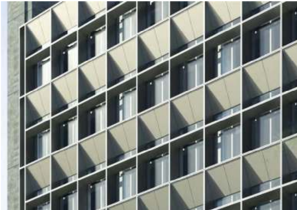
FIGURE 2: THIS IMAGE SHOWS THE GLAZED ALUMINUM CURTAINWALLS WITH ALUMINUM PANELING. THIS RENDERING IS COURTESY OF TURNER CONSTRUCTION.
